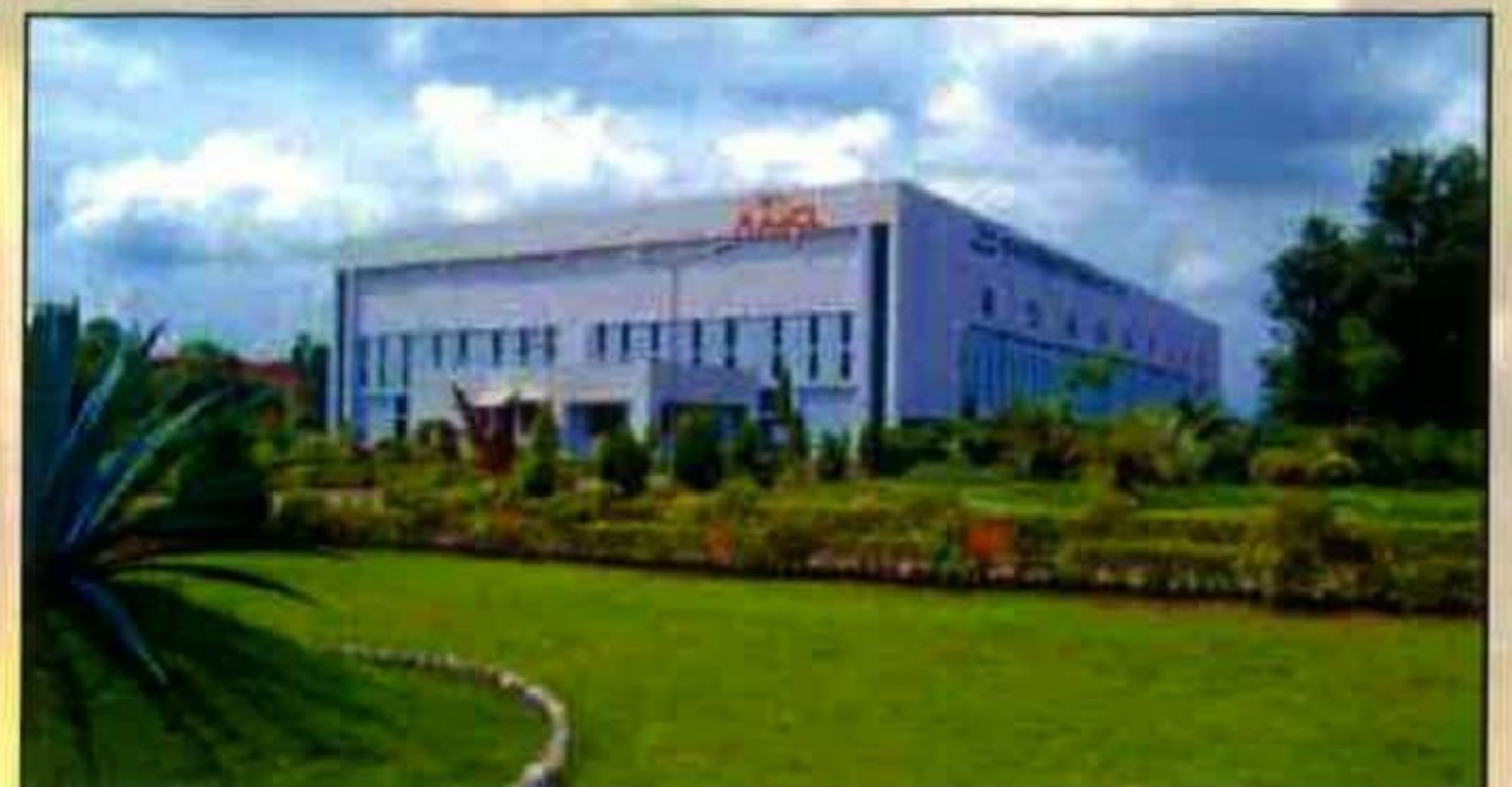
Works at Nagpur
